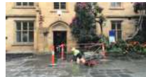
The works never stop on campus.
