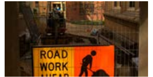
More construction. Old Arts.
